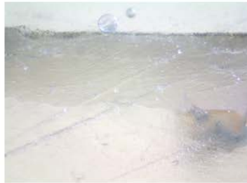
Visible light; before testing
